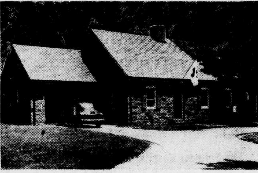
This is an exterior view of the Park Police substation at Military road and Beach drive in which the Red Cross fire-aid unit was formally established yesterday. —Star Staff Photos.
