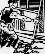
To determine the size of the storm sash measure one light of giass and give as the measurements and number of lights in up-per and lower sash.
