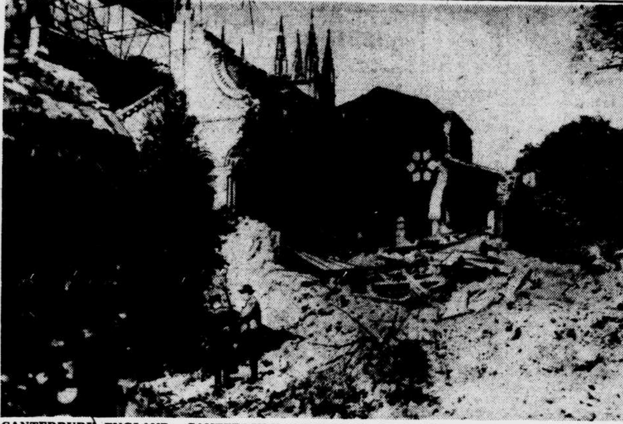
CANTERBURY, ENGLAND.—CANTERBURY CATHEDRAL DAMAGED BY BOMBS—Debris from the wrecked library of Canterbury Cathedral—cradle of the Anglican Church—is piled high after a German "blitz" on Canterbury. Rising in the background are spires of the main structure of the cathedral, which escaped a direct hit. Nazi planes attacked the city June 1. —A. P. Wirephoto.
