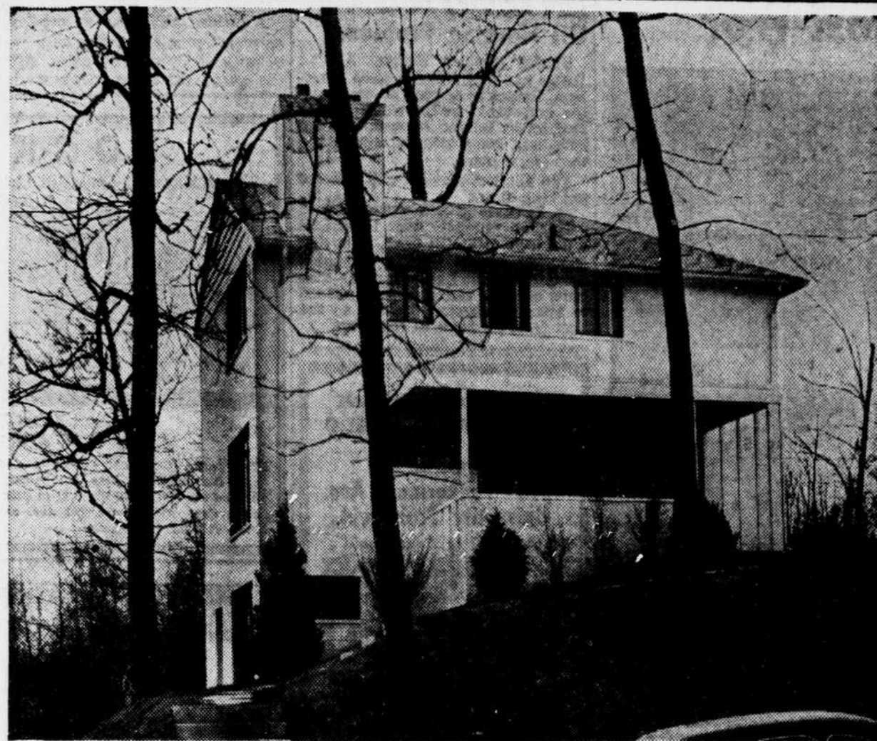
MONTICELLO ESTATES—Mr. and Mrs. E. J. McIntosh bought this new home at 2908 Argyle drive, Alexandria, Va., from the Monticello Development Corp. through the office of J. Garrett Beitzell. —Star Staff Photo.
