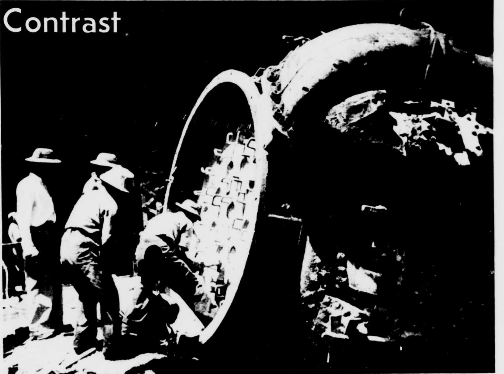
Graduate engineering trainees working on one of the Bessemer converters at the Indian steel plant of Tatas, pioneers of Indian heavy industry.
