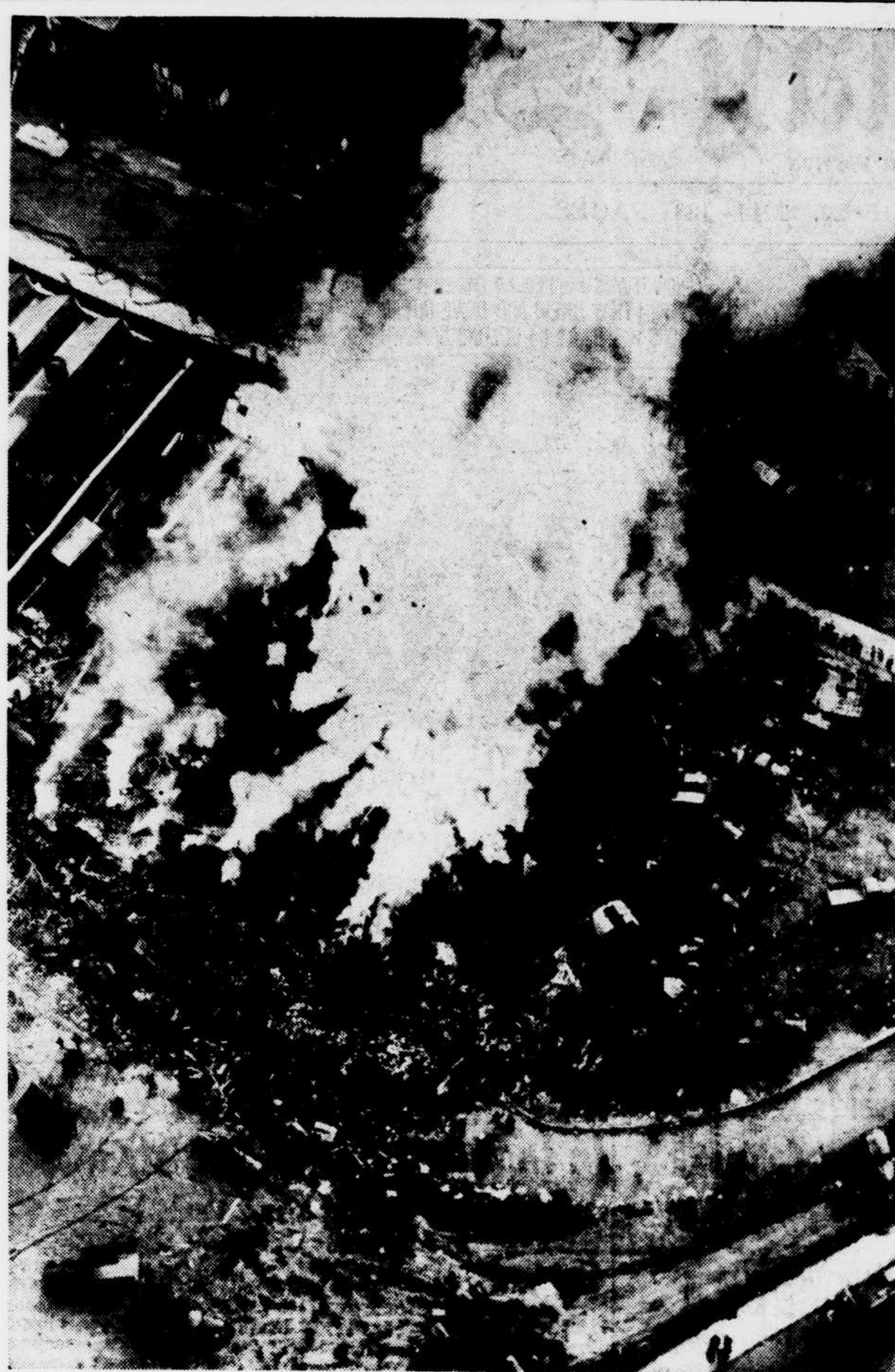
BRIDGEPORT, CONN.—EXPLOSION WRECKS ARSENAL—Six persons were missing last night after a series of explosions and fires ruined a brick building of the Remington Arms Co. plant here, one of the East's vital arsenals of war production. More than 25 others were injured. —A. P. Wirephoto.
