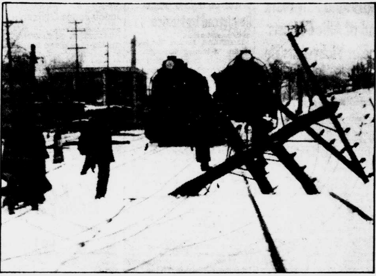
PITTSBURGH—An 18-inch snowfall, the heaviest in Pittsburgh's history, yesterday caused this snow-burdened power pole to collapse on the railroad tracks. Workmen with saws and axes removed it. The snowfall was blamed for four deaths, paralyzed traffic and hampered production of many steel mills and other factories busy on defense work.
