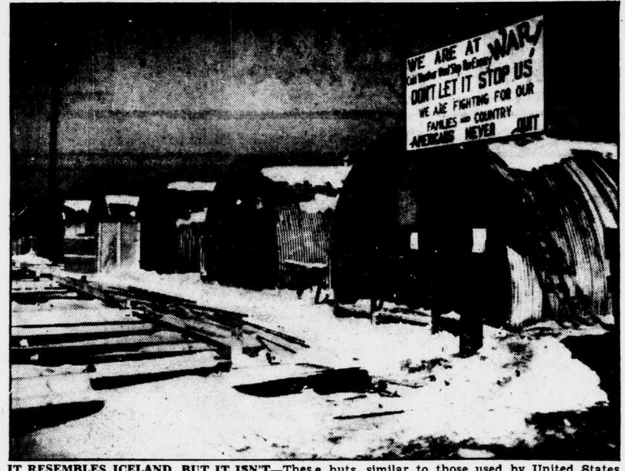
IT RESEMBLES ICELAND, BUT IT ISN'T—These huts, similar to those used by United States forces stationed in Iceland, were put up at Norfolk, Va., to house the expanding personnel of the Naval Training Station. A bit of snow added a atmosphere. Note the sign.
