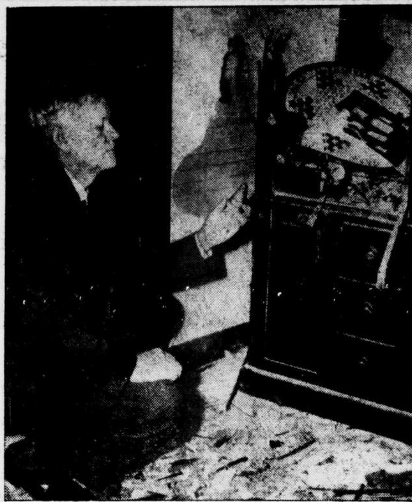
LONG BEACH, CALIF.—BARRAGE LEAVES MARK. —Dr. F. W. Stewart views damage done to his kitchen by an anti-aircraft shell, fired during the barrage sent up early yesterday. The shell failed to explode in the air and burst only after it had penetrated the roof of the kitchen and struck the floor.
