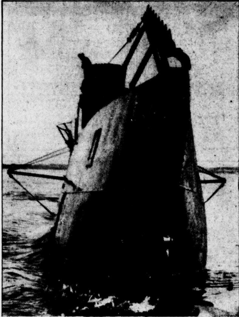
The row of sawteeth on the top of the bow of this German submarine is used to cut steel underwater nets.
