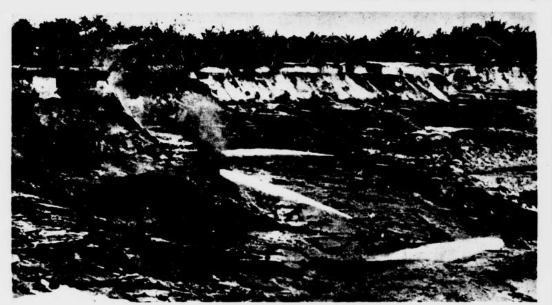
Sumatra, closest to the Japanese thrust against the Dutch Indies, is the source of most of their tin production, of which they produced 27 per cent of the world's supply last year. Most of the tin is mined by this process of washing the clay banks with high-pressure hoses, the resultant wash then being worked for the tin it contains
