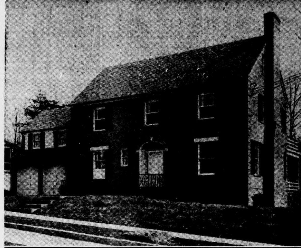
HOME IN KENT—This large dwelling at 5032 Glenbrook terrace N.W. was built for Mr. and Mrs. Herbert Budlong by C. D. Hobbs. Harvey Baxter designed it.
