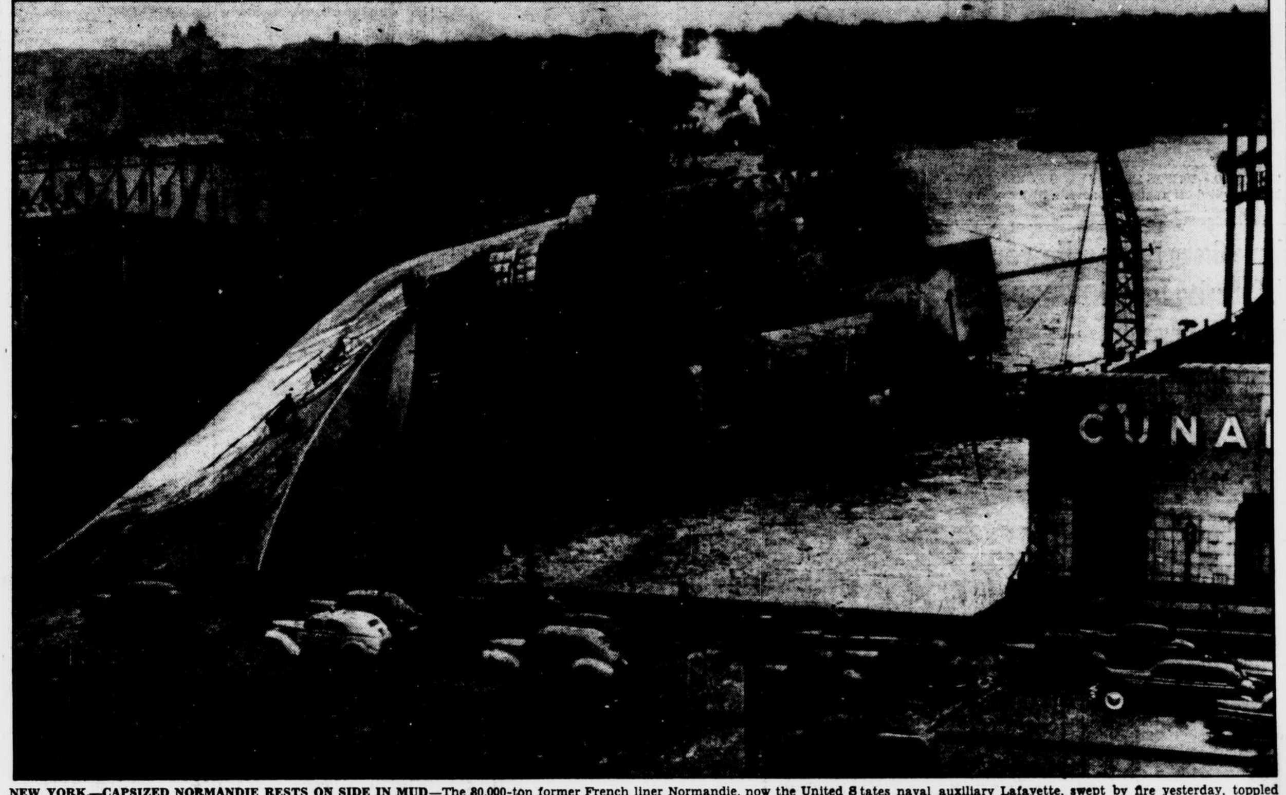
NEW YORK.—CAPSIZED NORMANDIE RESTS ON SIDE IN MUD —The 80,000-ton former French liner Normandie, now the United States naval auxiliary Lafayette, swept by fire yesterday, toppled over on her port side at her Hudson River pier today and came to rest in mud. Salvage experts expressed the opinion the capsized vessel could be righted in two or three months. (Story on Page A-3.) —A. P. Wirephoto.
