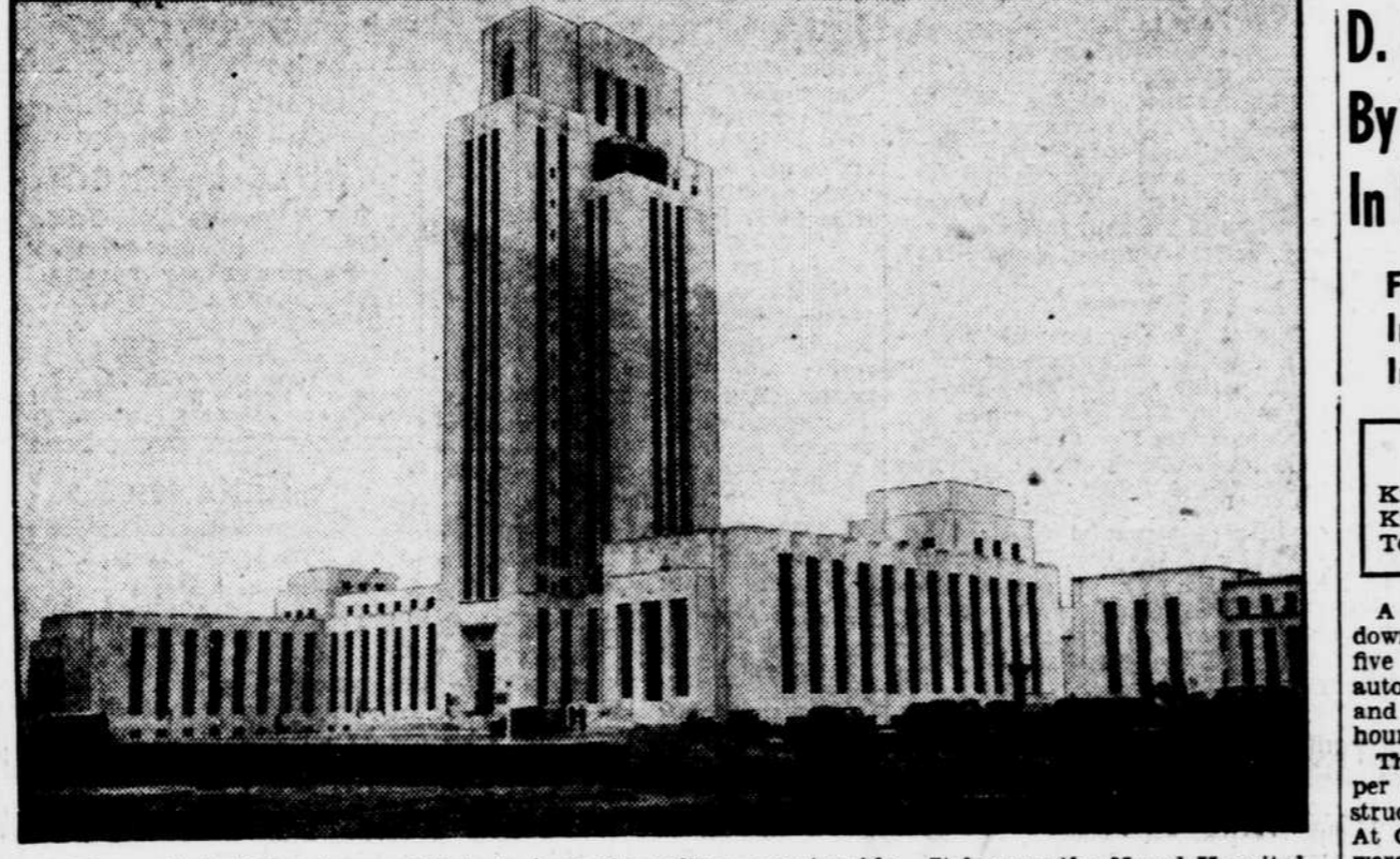
The main building towers 270 feet above the rolling countryside. It houses the Naval Hospital, Naval Medical School and Naval Dental School. Construction is of steel faced with pre-cast concrete aggregate panels.
