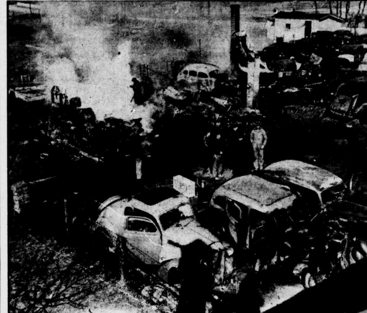
FIRE DESTROYS GARAGE, TIRES, AUTOS—An explosion in a heater today started a $10,000 fire which destroyed a garage, a small one-story house, 100 tires and 10 old automobiles at Groveton, Va., on highway No. 1, about 2 1/2 miles south of Alexandria. The property was owned by David S. Crockett.
