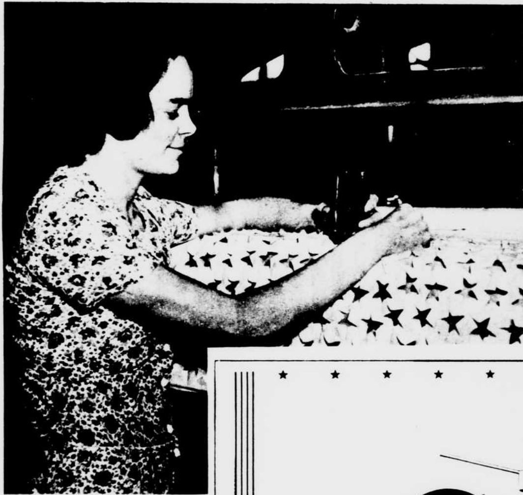
In this process Elizabeth O'Malley is dieing out the stars with a special cutter as she makes a stencil for applying stars to a flag. Thus a flag factory does its coloring and printing as well as its cutting and stitching in producing flags.
