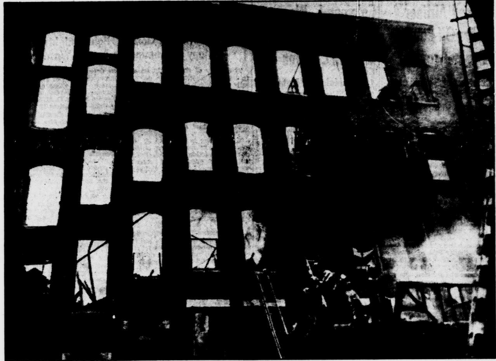
LYNN, MASS.—WHERE FLAMES TOOK HIGH TOLL—Only the walls were left standing after flames swept the Melvin Hall apartment house in downtown Lynn early today, taking a high toll of lives and injuring scores.
