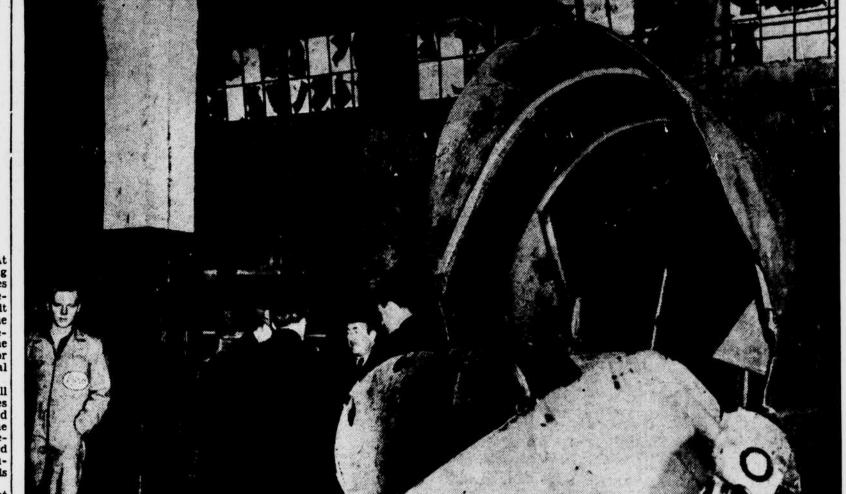
WRECKAGE OF TRUCK BLAST—Gasoline fumes, ignited by an acetylene torch, yesterday blasted this huge tank trailer out of shape, killing Wren Carlisle, welding company foreman, and virtually wrecking the interior of a workshop at Thirty-first and K streets N.W. Lawrence Carlisle (left), son of the man killed, works at a nearby filling station. Coroner A. Magruder MacDonald (center) came to the scene to investigate the -Star Staff Photo.
