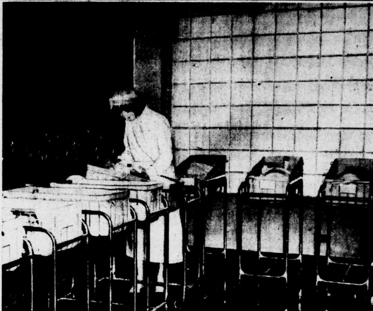
BLACKOUT PROBLEM SOLVED —Because of its modern design, Doctors' Hospital faced a special situation when planning air-raid precautions—large expanses of glass brick walls. This view of the nursery shows cribs lining the once translucent wall, now completely blacked out through use of aluminum paint. Full illumination may be used in the room.
