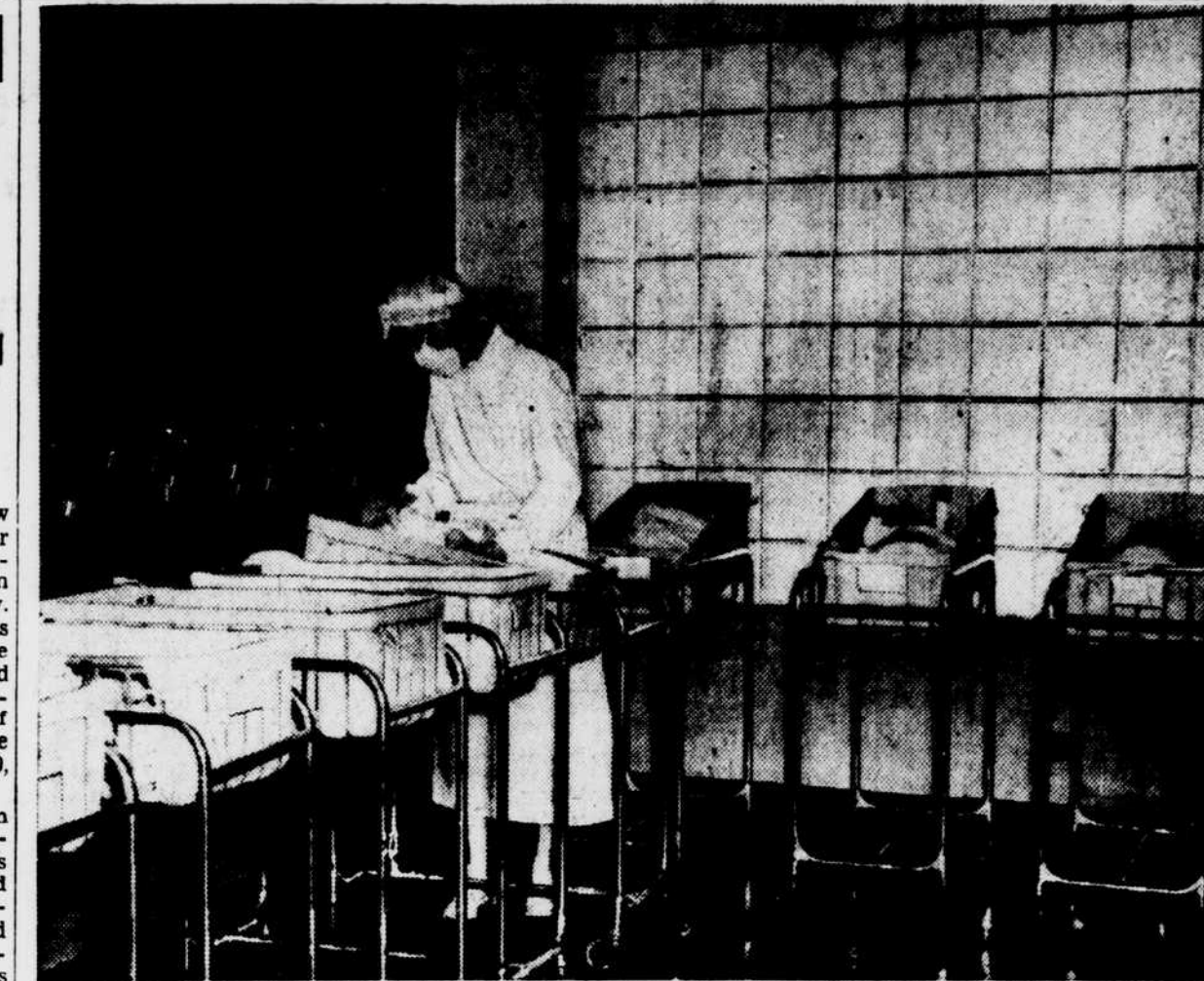
BLACKOUT PROBLEM SOLVED —Because of its modern design, Doctors' Hospital faced a special situation when planning air-raid precautions—large expanses of glass brick walls. This view of the nursery shows cribs lining the once translucent wall, now completely blacked out through use of aluminum paint. Full illumination may be used in the room.
