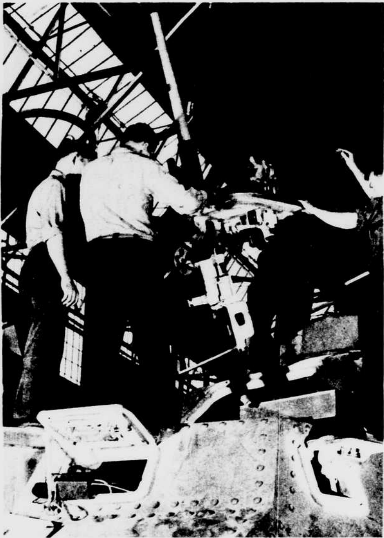
← Fully assembled, this 37 mm. anti-aircraft gun, carried to the tank by overhead crane, is being installed in an M-3. It carries a 75 mm. gun in the lower turret.
