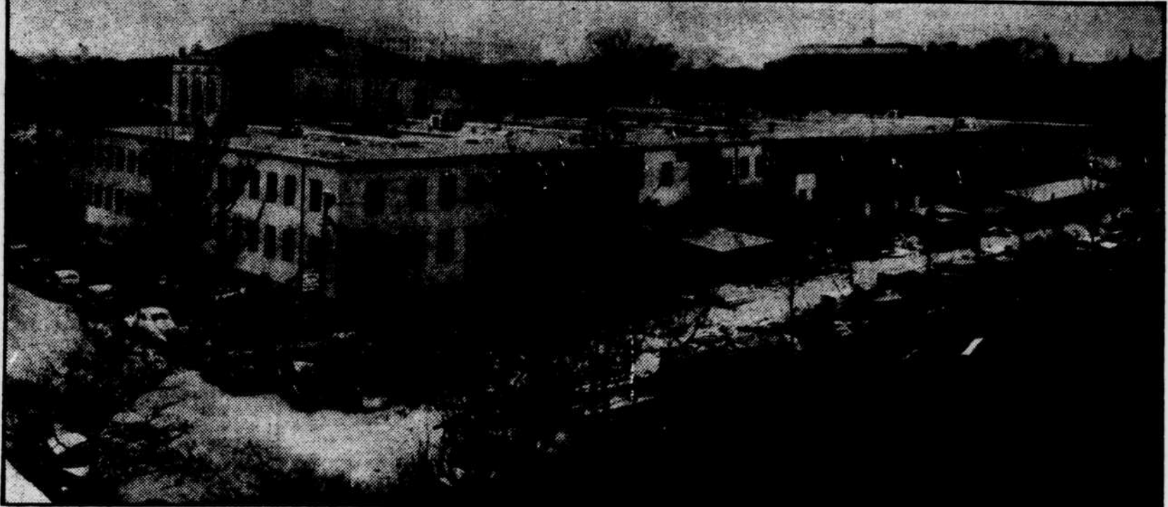
TEMPORARY BUILDING NEARLY READY—General view is given of Temporary Building S at Sixth street and Jefferson drive, which will be ready for occupancy January 15, a month ahead of schedule. This structure will add 120,000 square feet of office space, according to officials of the Ross Engineering Co. contractors. With six wings, the building will be 477 feet long and will cost $600,000 under contract by the Public Buildings Administration.
