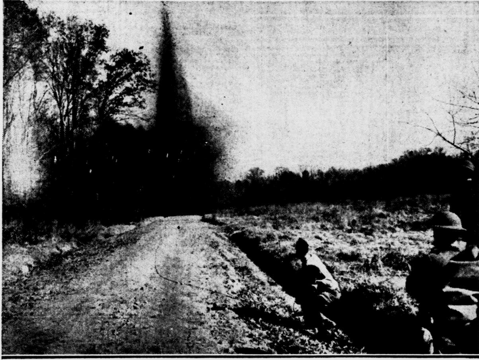
AND THEY DON'T REPLACE THE DIVOTS—The engineers are charged with the job of blowing up impediments created by the enemy and with demolishing roads and bridges that might be of use to the enemy. Therefore, all the selectees who go through the engineer training course at Fort Belvoir have to learn to handle explosives. Above, a selectee explosive charge is set off to blast a crater in a road.
