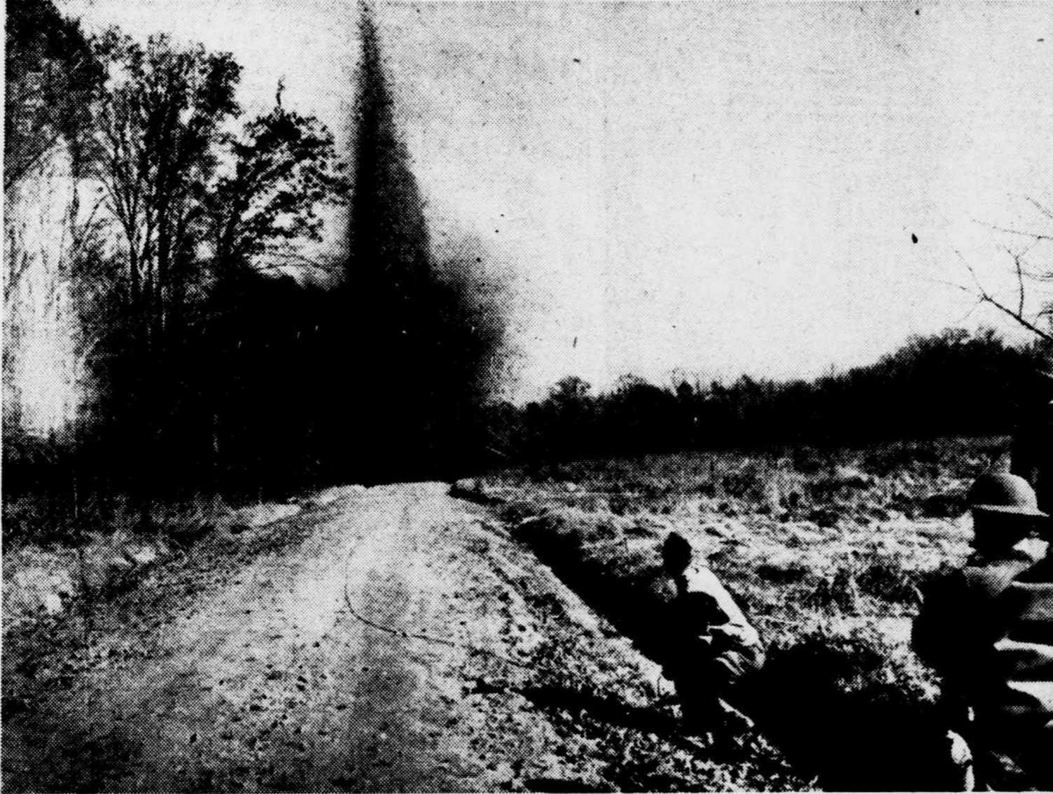
AND THEY DON'T REPLACE THE DIVOTS—The engineers are charged with the job of blowing up impediments created by the enemy and with demolishing roads and bridges that might be of use to the enemy. Therefore, all the selectees who go through the engineer training course at Fort Belvoir have to learn to handle explosives. Above, a heavy explosive charge is set off to blast a crater in a road.
