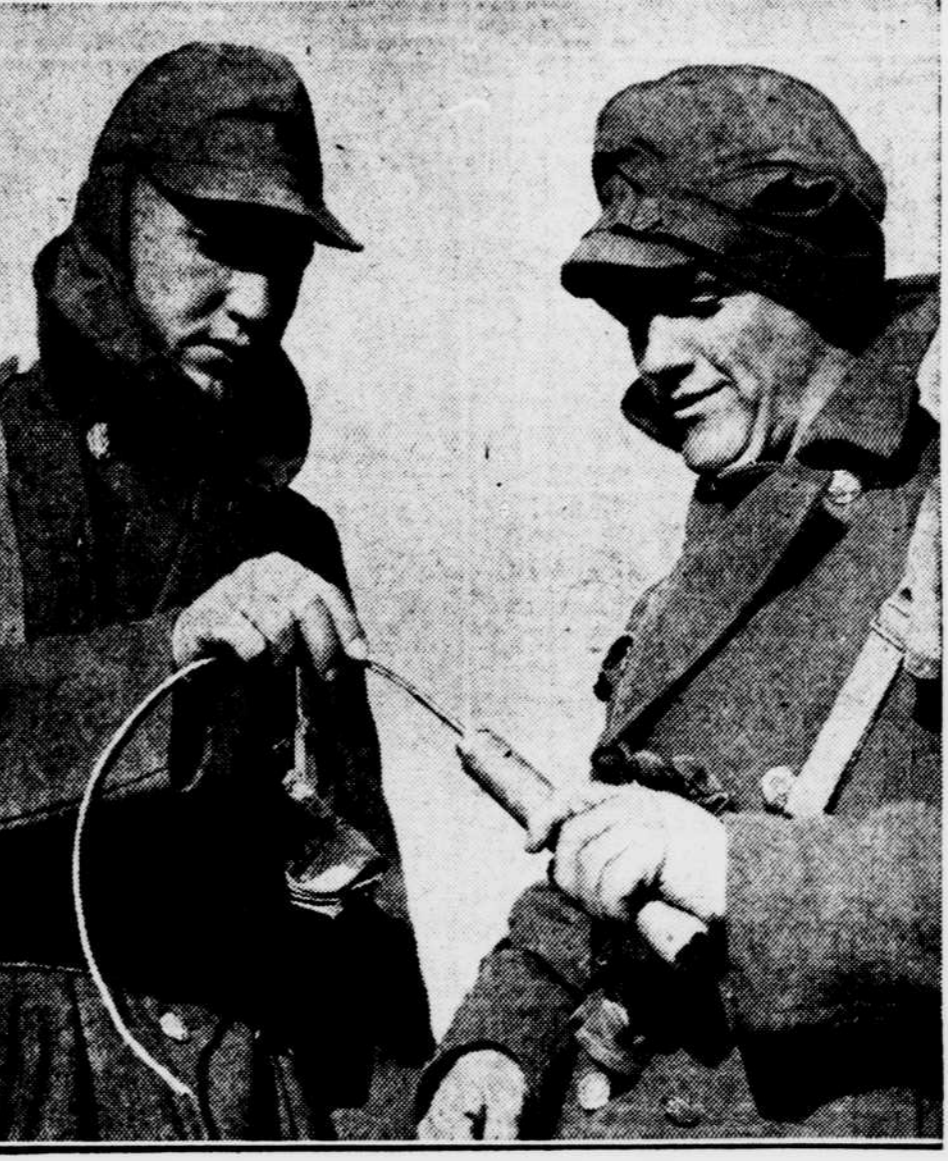
Every selectee is handed a charge of dynamite, with fuse, cap and assorted parts and required to set it off. Here Pvt. Fred Jenkins (left) and Pvt. Roscoe Rogers slip fuse into dynamite stick.
