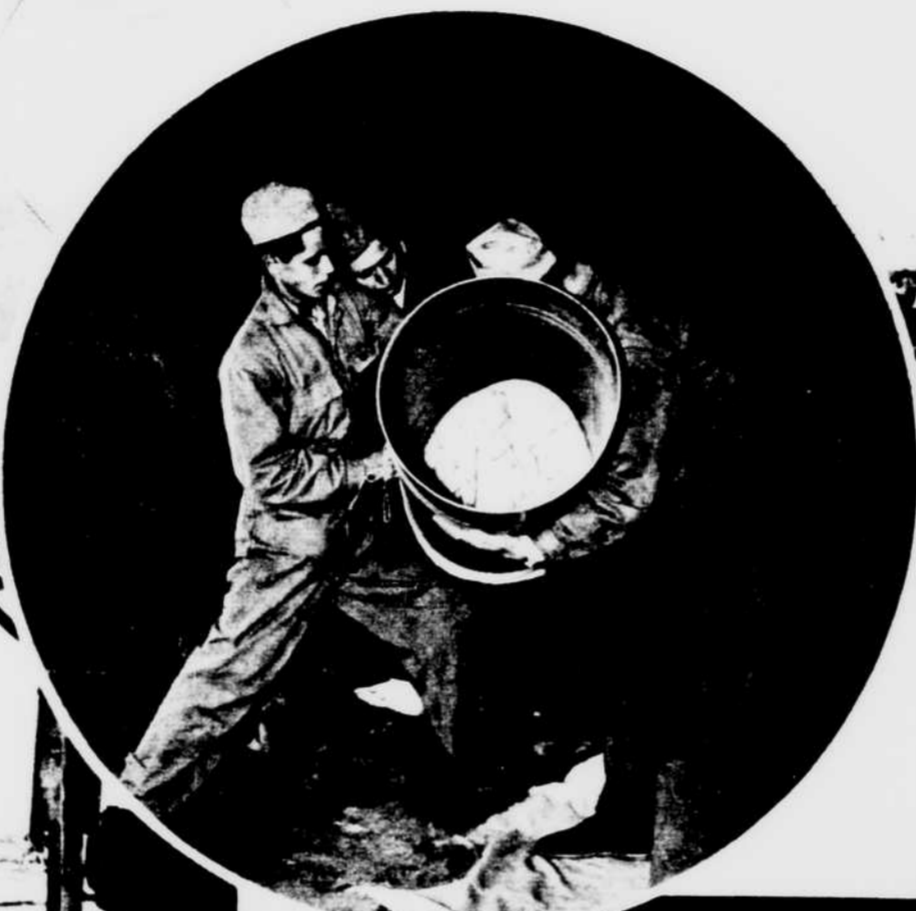
One of the tricks of stabilizing a balloon. This wind scoop is put into the lower stabilizer to fill it with air and prevent rolling or capsizing while the bag is being inflated.
