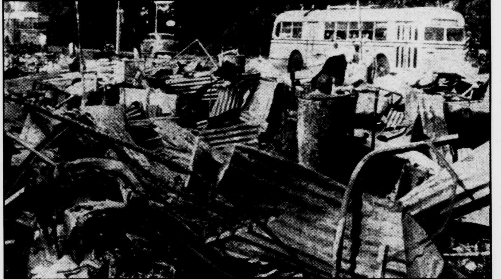
This twisted metal wreckage lay alongside a Honolulu street.
