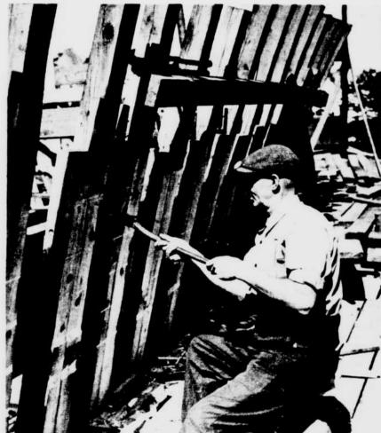
The adz, perhaps the oldest shipbuilding tool, is used by a master, Ansel Brewer. He is mortising the heavy ribs of a mine sweeper.
