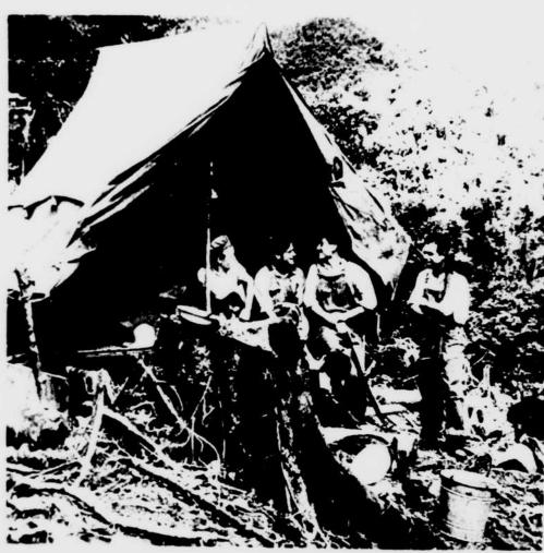
One of the first things the colony built was shelter for a saw mill. Since the mill was yet to be set up, there was no finished lumber for this job. Small trees cut from the forest form the crude framework.
