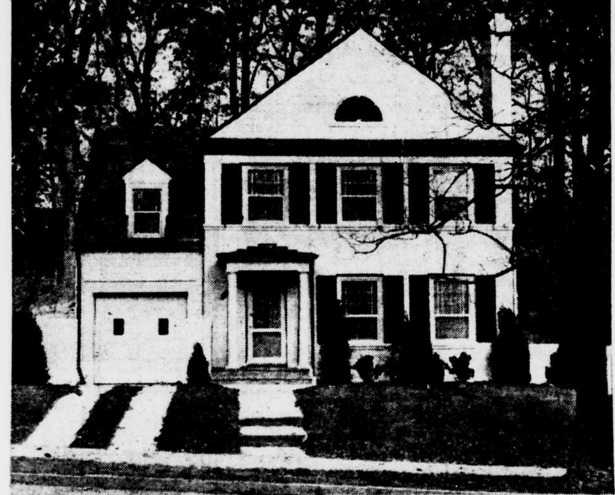
CLEVELAND PARK HOME —Mr. and Mrs. Warren Irbin bought the above house at 3077 Cleveland avenue N.W. from Barkley Bros., builders, through the office of the Thomas J. Fisher Co.
