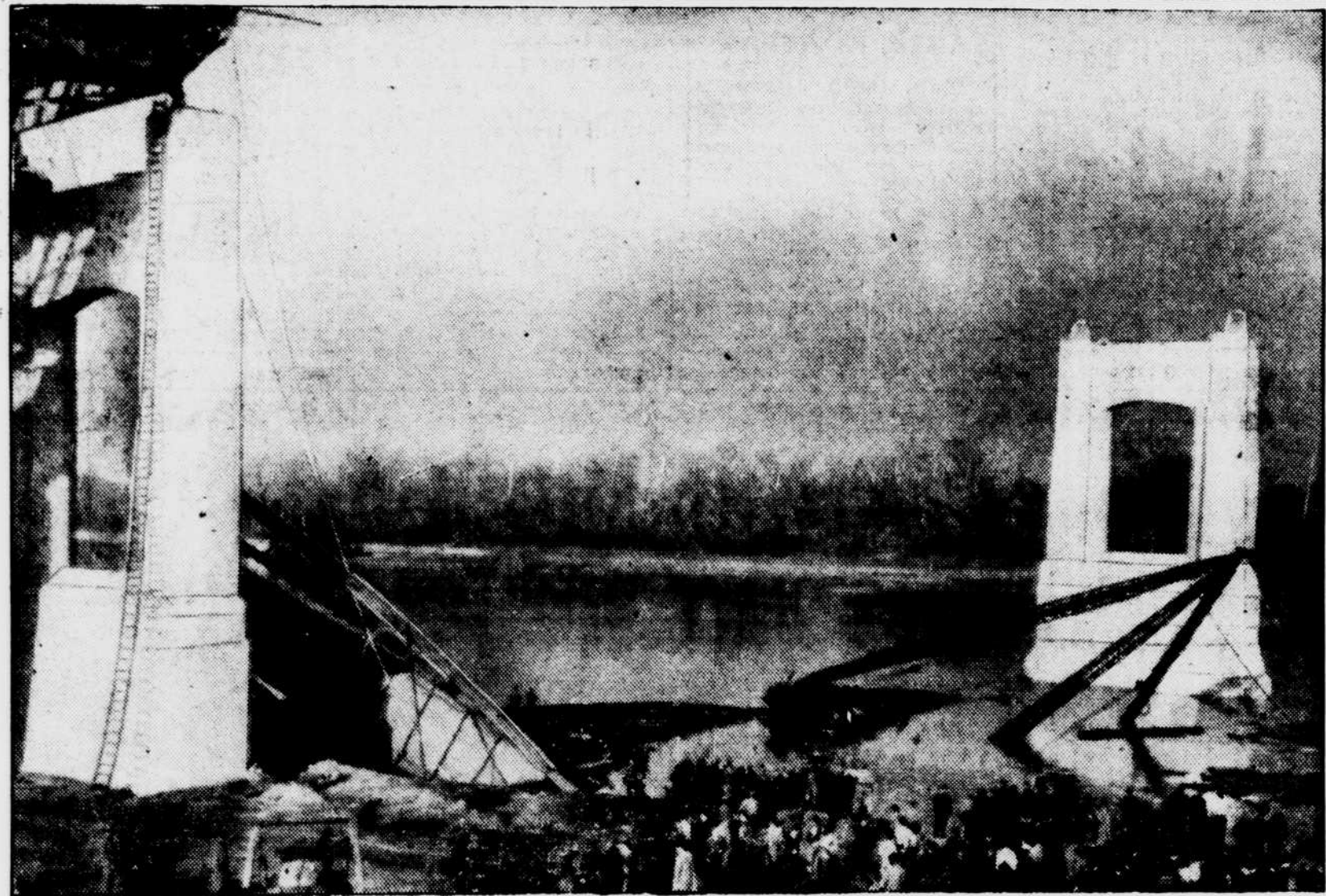
HARTFORD, CONN.—BRIDGE COLLAPSE KILLS EIGHT, SIX MISSING —At least eight workmen were killed and six are still missing after the new $1,900,000 Connecticut River Bridge collapsed as the final span was being lifted into place yesterday
