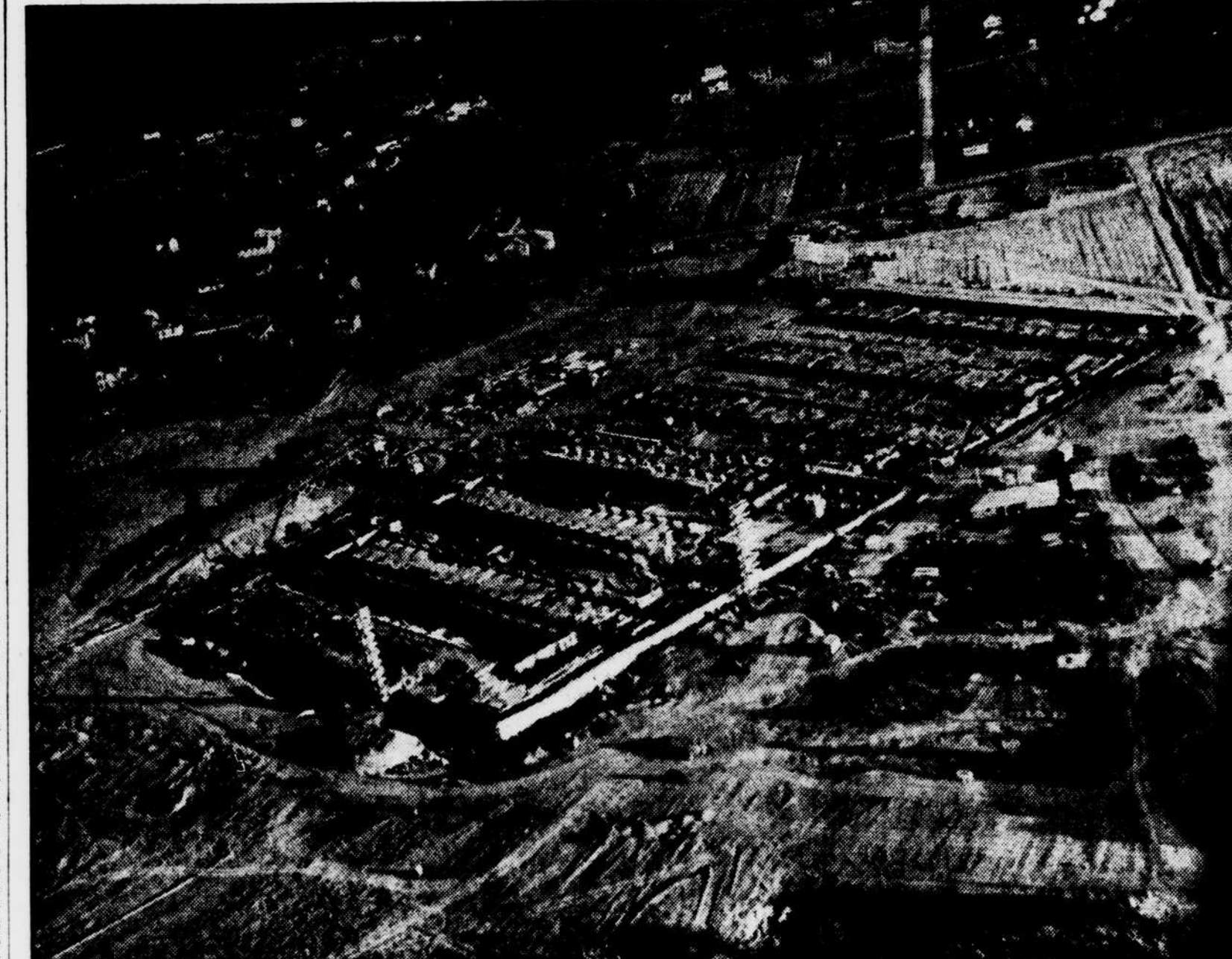
NEW FEDERAL OFFICE BUILDING RISING AT SUTTLAND, MD.—This air view of Federal Office Building No. 3 at Suttland, Md., looking southeast, shows progress of construction on the $4,100,000 project scheduled for completion next spring. The Silver Hill road crosses the picture beyond the 430-acre building site and the Suttland School can be seen in the center background facing the road. The Suttland road intersects from the left. The building will house about 4,500 workers and is about 6 miles from the Capitol. The Washington Suburban Sanitary Commission is selling a bond issue to provide funds for water and sewer facilities and special zoning powers have been granted Prince Georges County commissioners to protect the area. It has not been decided what officers will occupy the building. —Photo by Bill Young.
