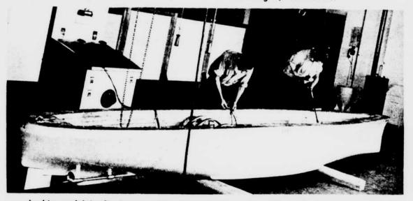
A ship model in final preparation for a tank test. All mechanism is tested and adjusted before the model is placed in the water.
