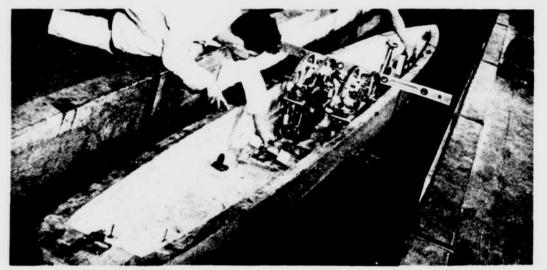
Ballasting the model to bring it to the proper waterline before making a selfpropulsion test under the towing carriage.
