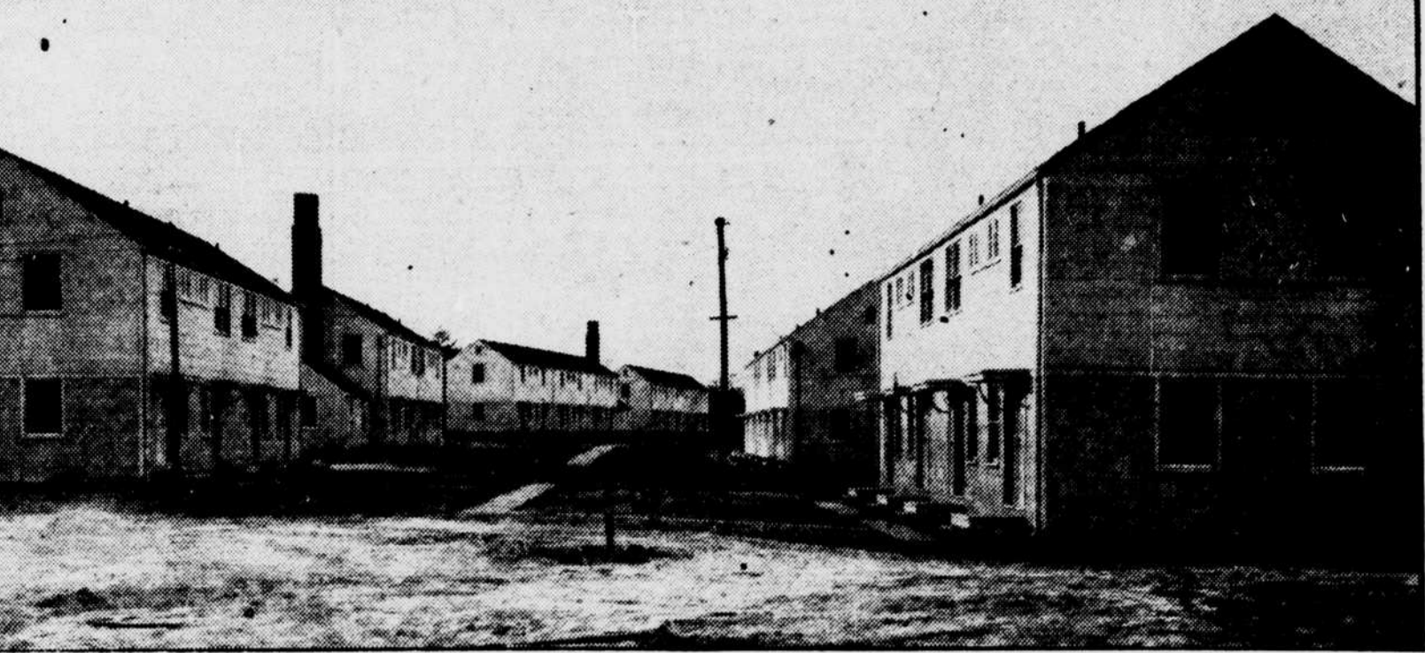
NEW HOUSES FOR DEFENSE WORKERS AT GREENBELT, MD.—These are some of the 1,000 new living units which are being completed for defense workers at Greenbelt, the Government's housing project. They were built of asbestos shingle over
