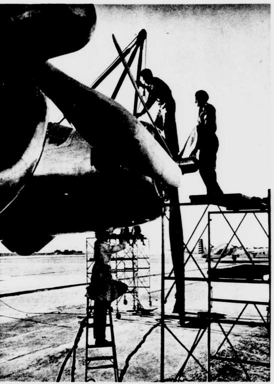
It's a tall job to check the B-19's four giant motors after a test flight. Compare the size of those propeller blades with the men working on one of the engines.
