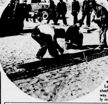
Laying the first section of steel strips to start the runway. Each strip hooks tightly into the other.
