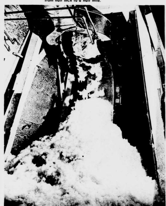
After its final washing, the finished, fluffy fiber drops into a "snow" mound, ready to be pressed into bales. In this form it is shipped to Canada and South America as well as to domestic users.
