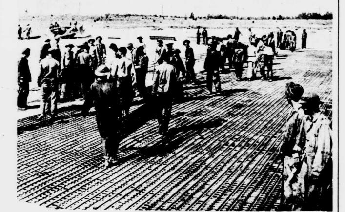
The two views above show how rapidly the laying of the great metal surface progresses after the bull-dozers have erased every hummock and swale. They were taken the day the first strips were laid.
