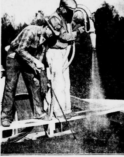
To carry out the process, John Sullivan holds the screen wire away from the rubberized, inflated balloon while "Tex" Bennett blows the nozzle-mixed concrete on for the first coat. The screen wire makes it possible for the balloon to be completely surrounded with concrete.
