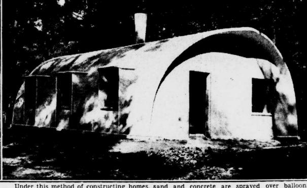
Under this method of constructing homes, sand and concrete are sprayed over balloons, which later are deflated. By using balloons of different shapes, some variety in the outside of the buildings can be obtained. Inside, the house shown here is divided into two bedrooms, a living room with fireplace, a kitchen and a bath.
