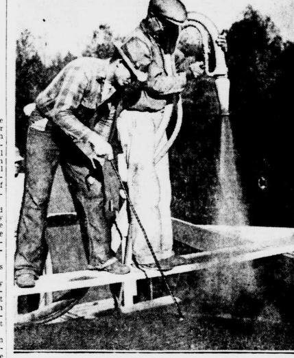
To carry out the process, John Sullivan holds the screen wire away from the rubberized, inflated balloon while "Tex" Bennett blows the nozzle-mixed concrete on for the first coat. The screen wire makes it possible for the balloon to be completely surrounded with concrete.
