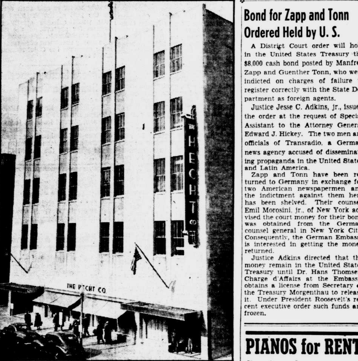
A view of the exterior of the seven-story structure, located on E street N.W., between Sixth and Seventh streets. The addition will provide a main entrance on E street.
