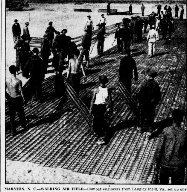
of the Army's newly-designed portable runways near here to enable planes engaged in the Carolina maneuvers to land on the treacherous, sandy terrain. Strips of metal grating 16 inches wide, 10 feet long and one-eighth of an inch thick are locked together, forming a landing area 150 feet wide and 3,000 feet long. -A. P. Photo.
