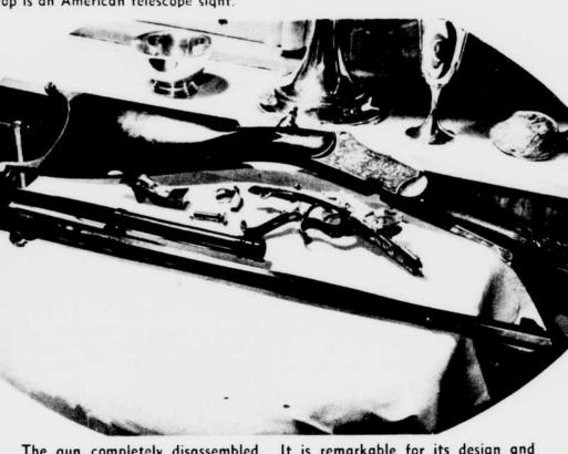
The gun completely disassembled. It is remarkable for its design and may be taken apart without the aid of tools by simply opening lugs and removing one thumb pin.
