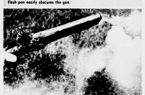
The action is completed. Recoil has raised the barrel several inches.
