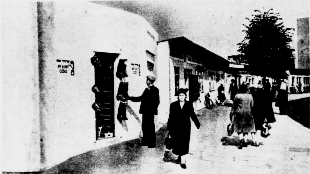
Another view of Coventry's resurrection. Some of the little one-story stores in the blasted area are of concrete, some merely of corrugated metal.
