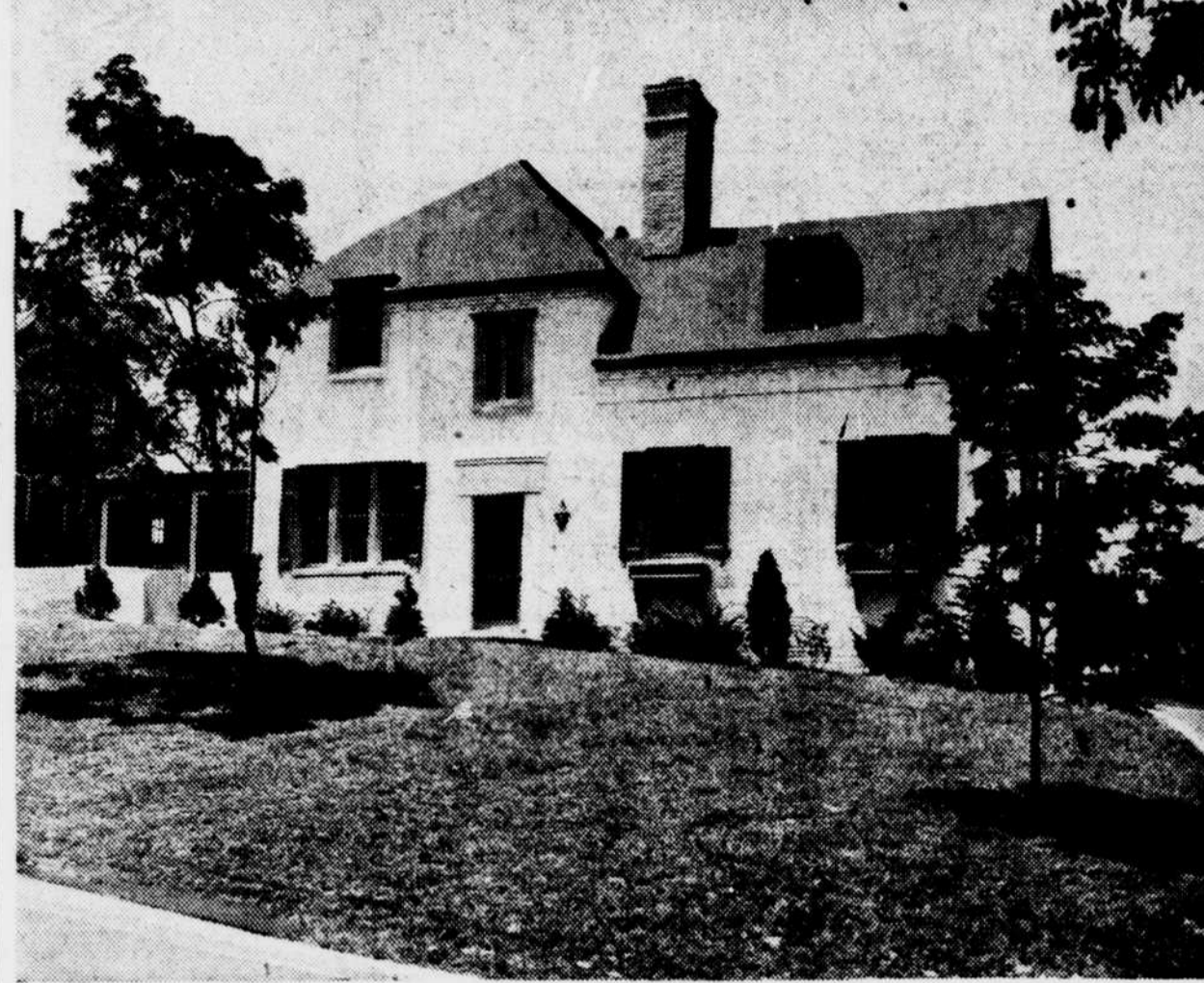
IN ARLINGTON—New home of Mr. and Mrs. Walter A. Brooks at 3214 North Woodrow street, Country Club Hills, Va., which was built by Behm & Beger, and sold through the office of K. D. Brumback. Louis R. Moss designed the house.
