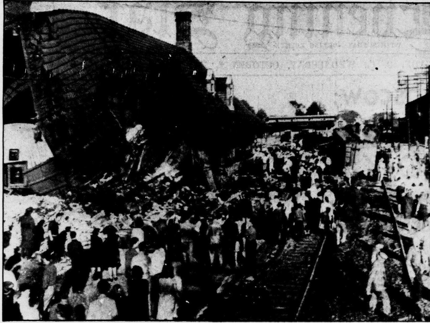
LANSING, MICH.—FAST FREIGHT HURTLER TRACK, WRECKS STATION—View of the wreckage of a Lansing depot after a fast freight leaped the tracks yesterday, whipping a string of cars in a destructive arc. The 50-car train, laden with fruit and other perishables, spilled much of its load over a three-block stretch.
