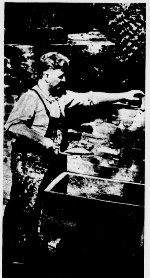
He lays bricks before breakfast and looks like a hewer and hauler
