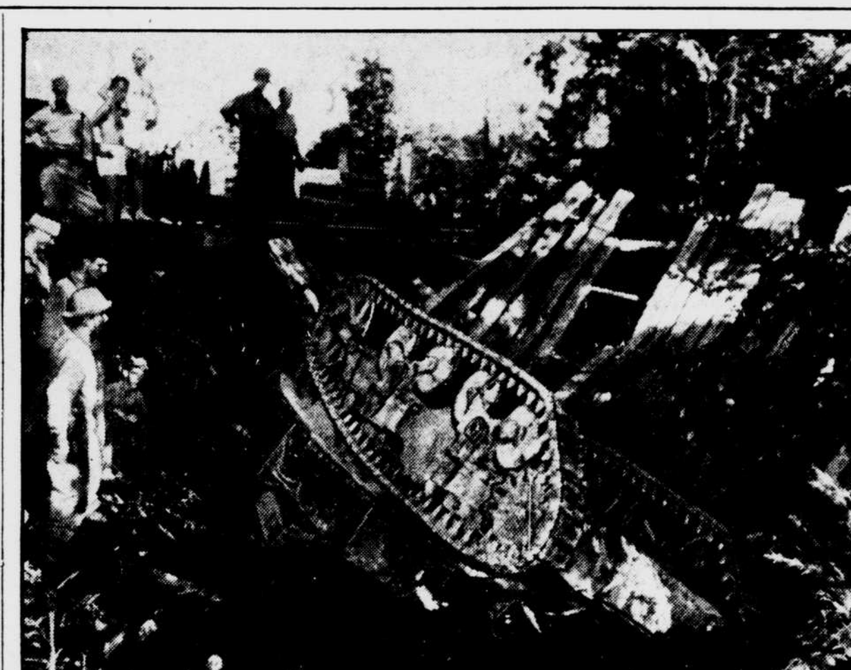
MANY, LA.—MANEUVERS MISHAP—Weakened by passage of other tanks, this bridge, over Lockwood Creek, near here, collapsed as a light tank was passing over during the "war" between the 2d and 3d Armies. None of the tank's crew was injured and the machine was rolling merrily along again within two hours.
