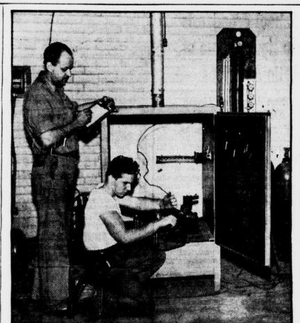
**REFRIGERATION REPAIR**—Under the eye of Instructor Ralph T. Midyette, Herbert Cole, student at the Chamberlain Vocational School, works on a refrigerator repair job. The shop also is equipped for air-conditioning repair and is said to be the only public vocational school with this equipment.
