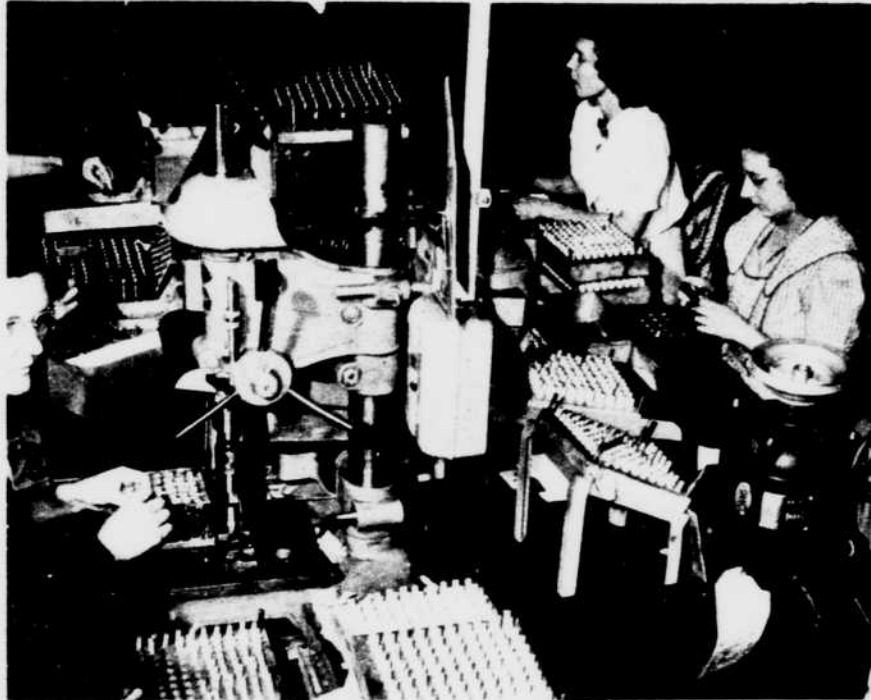
Women "spark" the aircraft defense program. The nimble fingers of hundreds of women workers are assembling a new type aviation spark plug at this Flint, Mich., plant.
