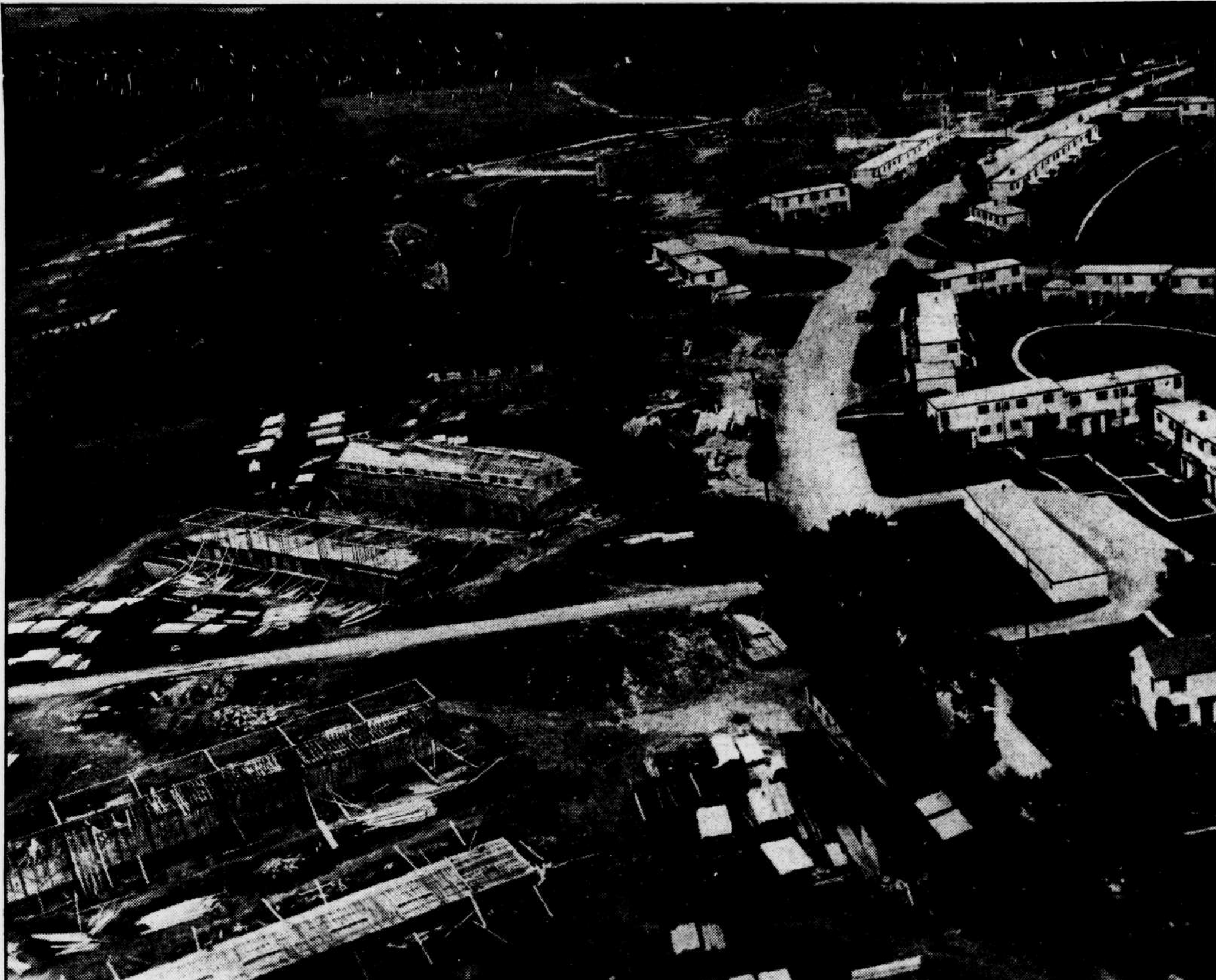
DEFENSE HOMES AT GREENBELT—This aerial photograph shows the progress being made on the 1,000-unit defense housing project for Federal workers at Greenbelt, Md. Work was begun August 8 under the supervision of the Farm Security Administration. Cost of the work is estimated in excess of $1,000,000.—Air View by George W. Young.
