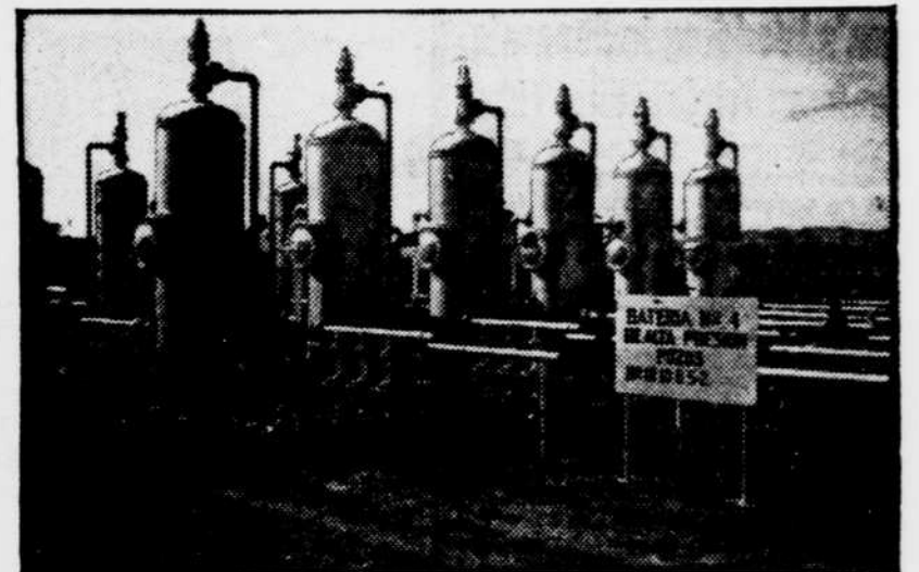
High pressure batteries at the Northern oil fields, Mexico.
