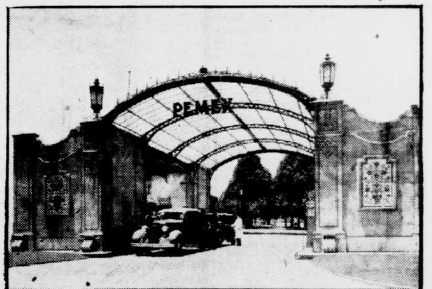
The type of urban service stations in Mexico City. Architecture is Mexican-Colonial. Modern, up-to-the-minute.
