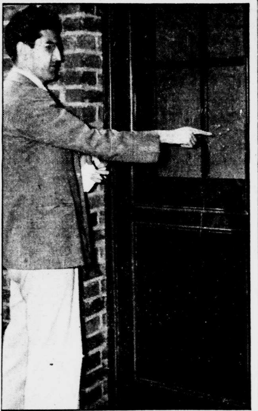
Through this back door of an apartment at 114 O street S.W., four bullets flew in quick succession yesterday to find their mark in the body of 15-year-old Ellen Cannon. Reporter points to holes in door made by bullets. —Star Staff Photos.
