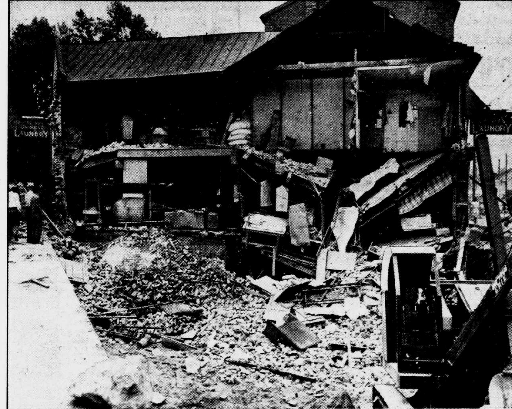
HALF OF BUILDING COLLAPSES —The entire side wall and half of the building in which Ting Moy runs a Chinese hand laundry, in the 1200 block of King street, Alexandria, Va., collapsed yesterday. Workers were digging a foundation for a new building next door when the wall collapsed. Two workers and a Chinese were slightly injured. Thousands of shirts and an unknown number of collars were buried in debris. Note objects still hanging on intact walls of the building. —Star Staff Photo.
