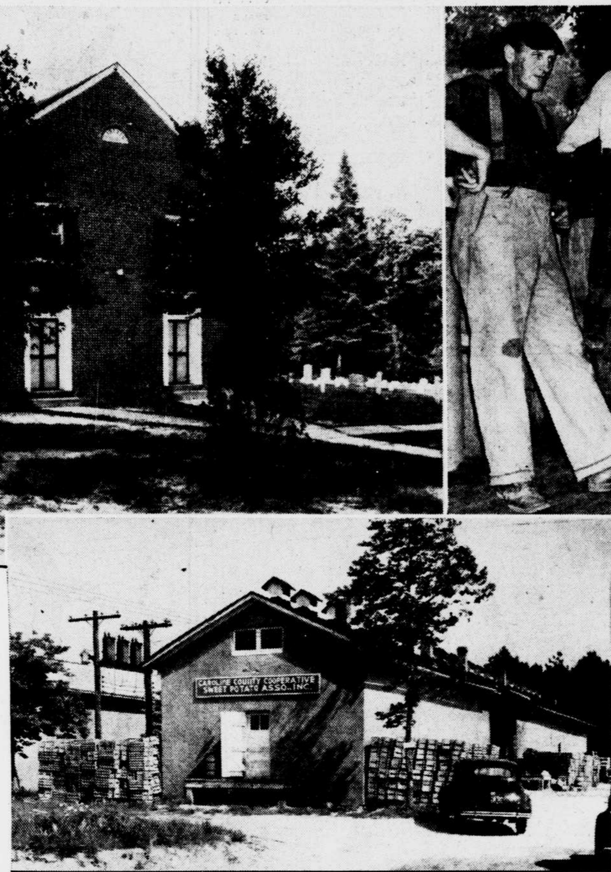
Here is one of the few businesses which must be abandoned—the sweet potato processing factory of the Caroline County Co-operative Sweet Potato Association, Inc. It has been in existence eight years and is described by its stockholders as a highly successful venture.
