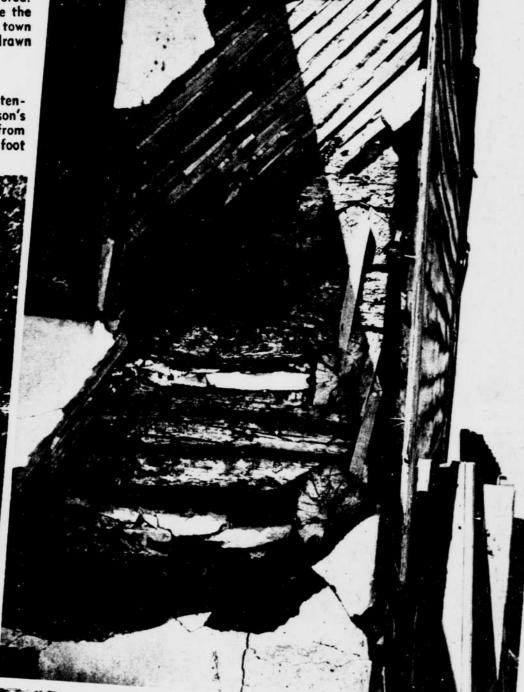
Made to last. Evidence that the early settlers built homes for posterity is found by examining the manner in which heavy hewn timbers were notched in place.
