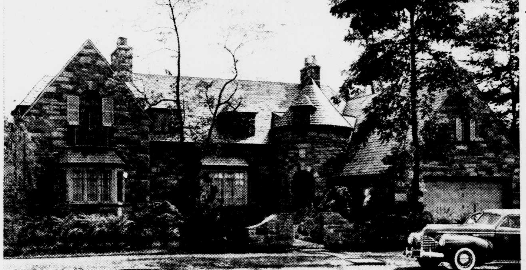
LARGE DWELLING COMPLETED —The new home of Mrs. Martha M. Bache at 4532 Macomb street N.W., which was built for her by Korzendorfer & Brooks and designed by V. T. H. Bien. —Star Staff Photos.
