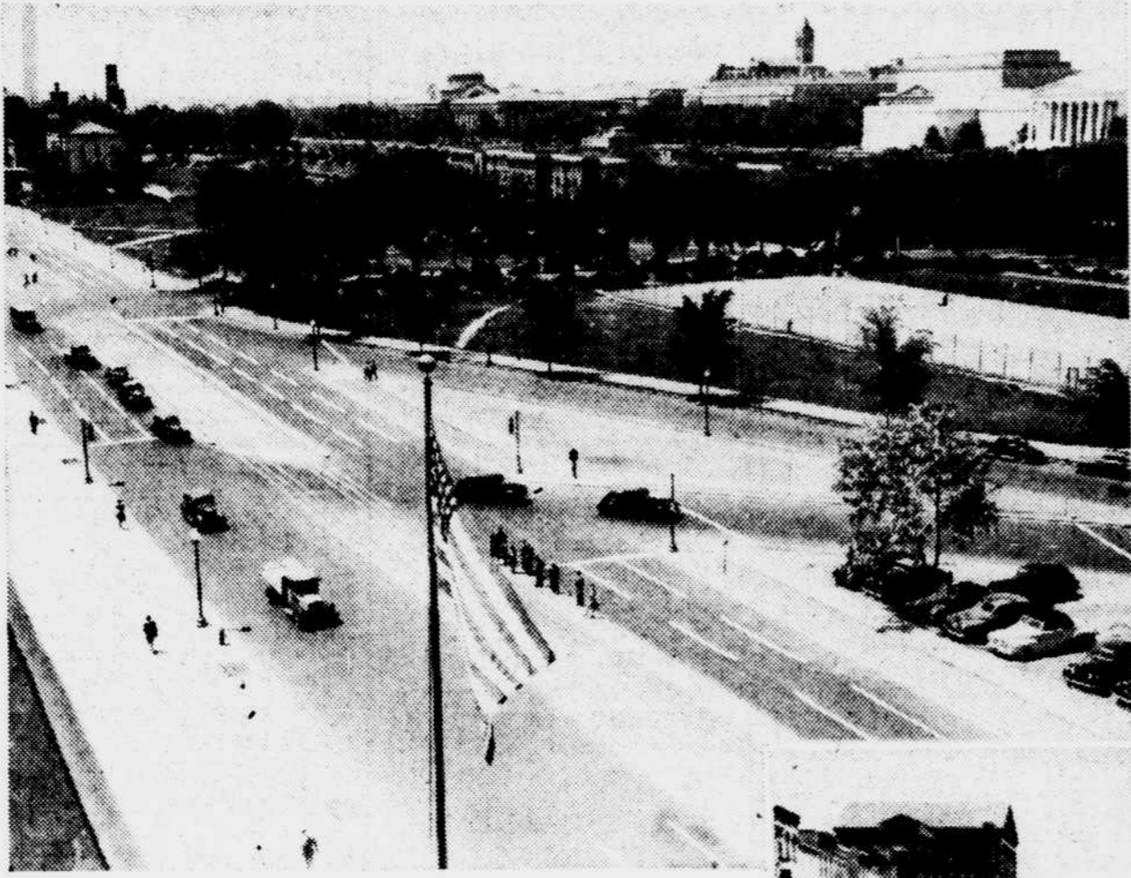
INTERLOCKED CHANGES ADVISED —Many improvements outside the highway program, but closely related, have been recommended to insure greater safety. One of these is modern channelization of streets on the pattern, as shown in this photo, of the intersection of Fourth street and Maryland and Independence avenues S.W.
