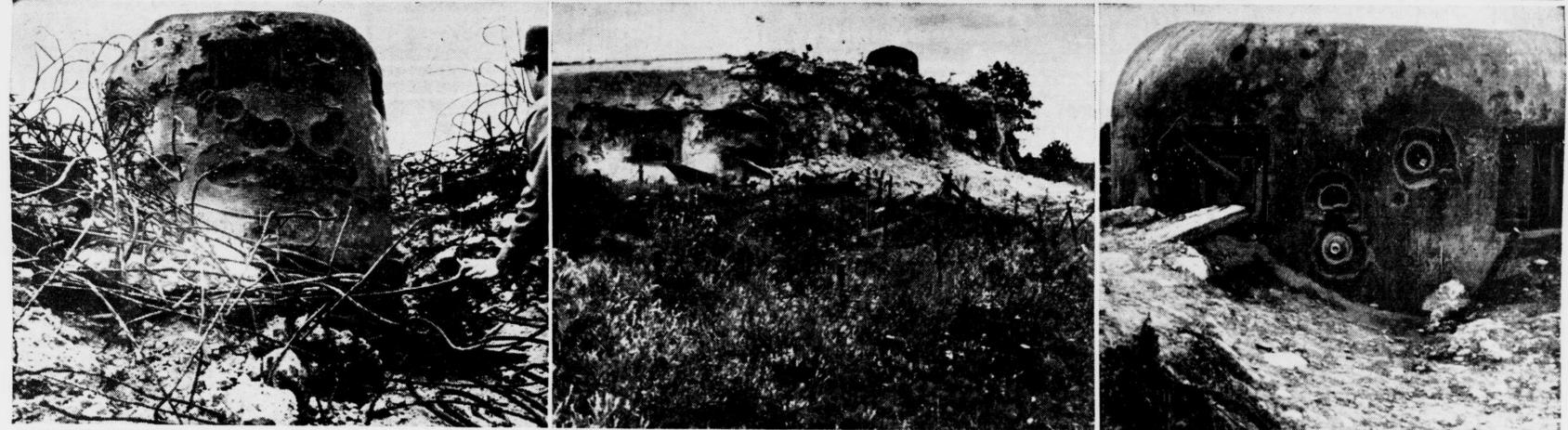
WHEN STEEL MEETS STEEL—This is an example of the damage done to the A casemate opposite Breisach, damaged by German guns firing from positions 200 yards Maginot Line forts in the May-June battles of 1940. Above is a pillbox away, across the Rhine. These pictures were obtained by the Chicago Tribune. opposite Breisach, Germany. The walls are of 12-inch steel.
