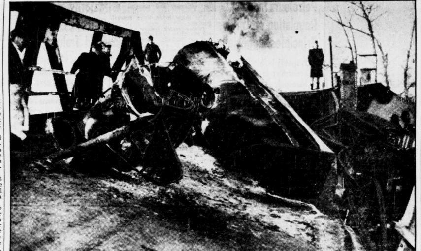
LE MARS, IOWA.-THE BRIDGE COULDN'T STAND THE HEAT -Terrific heat from a burning gasoline transport twisted the structure of this steel and concrete highway bridge near here
